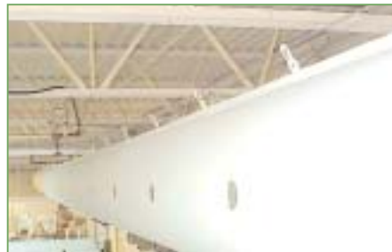
Wire cable and small duct clips make hanging fabric duct similar to hanging a shower curtain.
