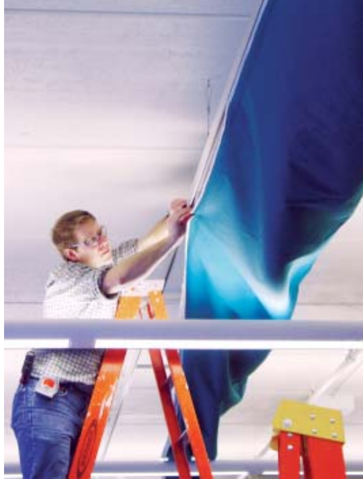
Fabric duct's light weight requires fewer workers to install compared to metal ductwork.
